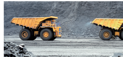
Mining construction site
